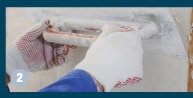
Immediately after mixing, apply the stucco with a metal spatula or plasterer's trowel, depending on the required effect.
